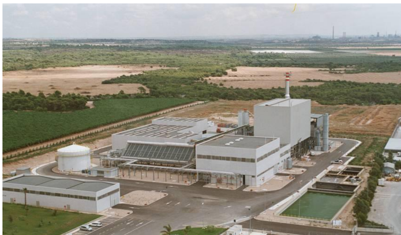
Figure 5. View of Massafra incinerator plant.
