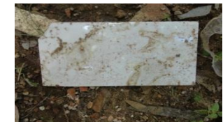
Broken Tiles Piece
