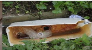
Damaged Sanitary Items
