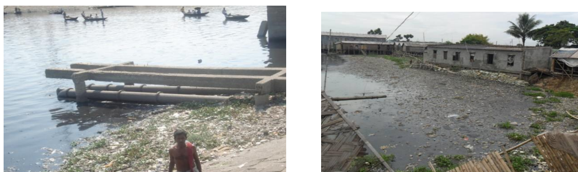
Figure 3 Industrial waste water falls into the river
