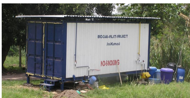
Figure 5: Second dry digester made of higher quality shipping container
