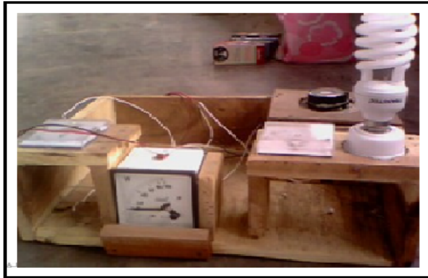
Figure.5: Measurement of power factor with capacitor.
