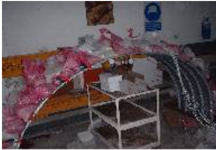
Fig. 7. Sand bag loading on cylindrical shell roofing
