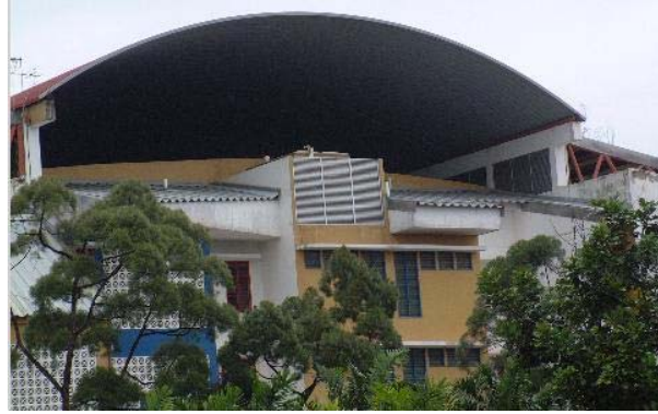
Fig. 5. Self-supporting roofing element at Universiti Putra Malaysia
