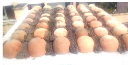
b) Mortar topping on and around mud pot
