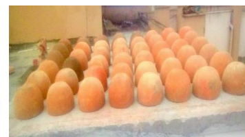
b) Mud pot on top roof slab
