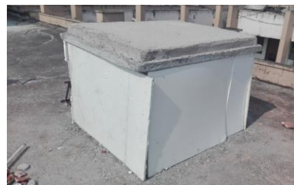
Fig.5: Side walls covered
