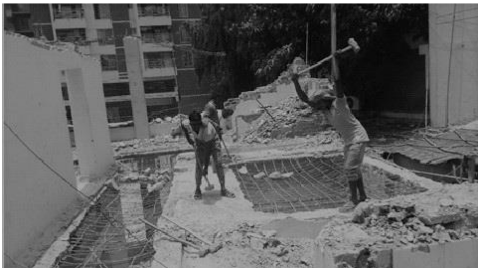
Fig. 2: Manual Deconstruction work in progress in Dhanmondi residential area, Dhaka
