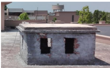
Fig.4: Side walls exposed
