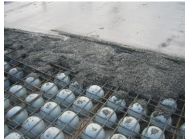
Fig.1: Bubble deck system (source: Canadian consulting engineer)
