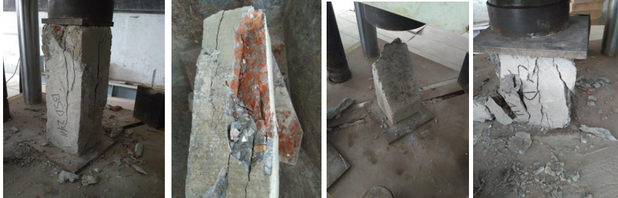
Fig.2: Monolithic failure (P); Fig.3: Substrate failure (P); Fig.4: Shear failure (P); Fig.5: monolithic failure (C);
