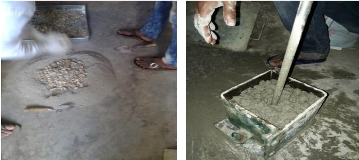
Fig. 7: Casting of concrete.
