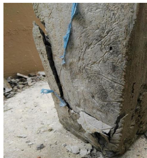
(b) Failure pattern for column containing 20% replacement of cement using ceramic waste powder
