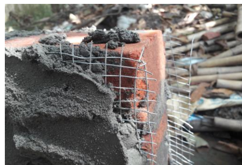
Fig. 4 Brick wall with ferrocement coating
