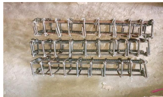
Fig. 8: Steel framework of RCC beam.
