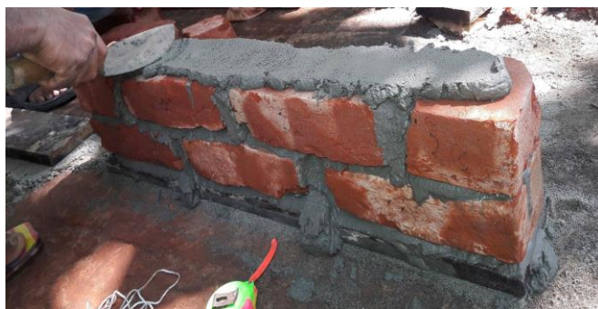
Fig. 3 Construction process of brick wall
