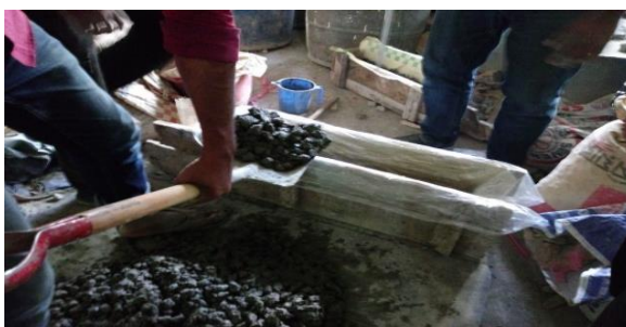
Fig. 9: RCC beam casting on prepared mould.
