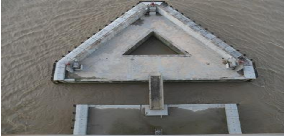
Figure 2: Basement of Bridge pier
