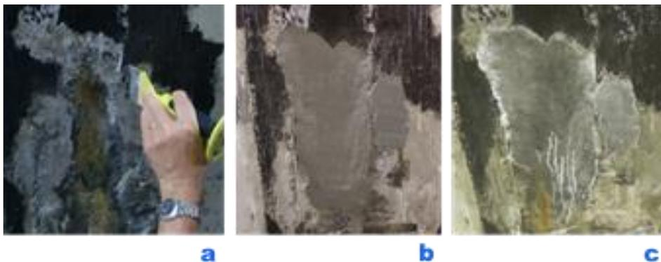
Figure 3. Self-healing mortar applied in practice: a) Surface preparations, b) Application, c) Visible limestone formation (white lines) on the surface of the set repair mortar [7]
