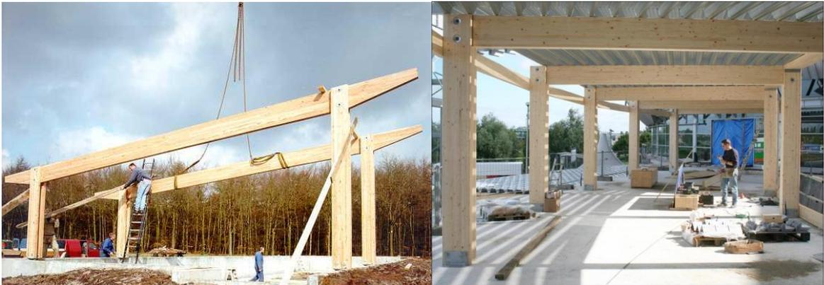
Fig. 10. Examples of timber frame buildings with two expanded tubes per moment transmitting connection having the same moment capacity as the glued laminated timber beams.
