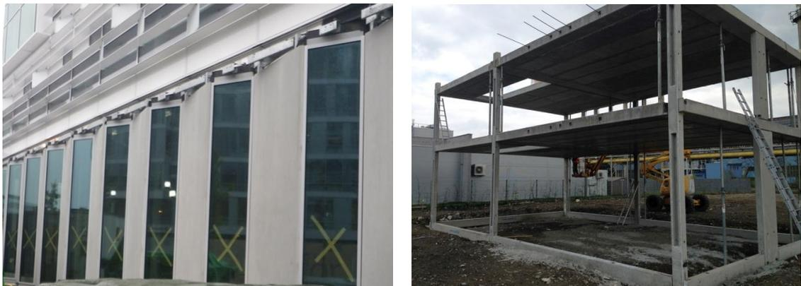
Fig 4 (a) external façade panels from textile reinforced UHPC, construction Skanska CZ, Malmö, Sweden (photo Skanska), (b) prototype of HPC subtle frame for residential buildings under construction in University Center for Energy Efficient Buildings
