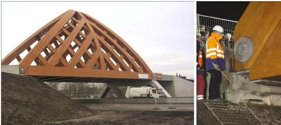
Fig. 6. Bridge at Sneek (NL) highest load category (left); Bridge support during erection stage (right).
