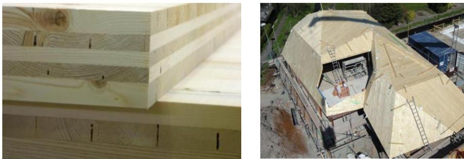
Fig. 8. Five layered Cross-Laminated-Wood (left); Application of CLT in a self-supporting roof (right).
