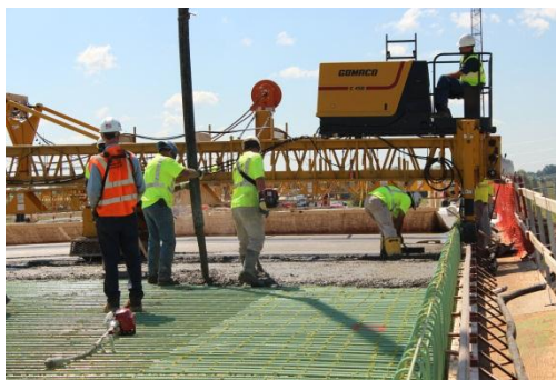
Figure 2: Concrete pouring and finishing work using screed machine
