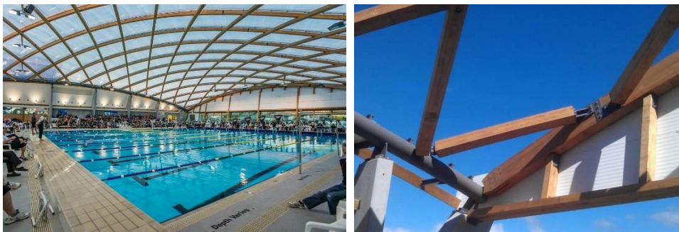
Figure 2: Coastland Aquatic Center (left), roof connections (right).
