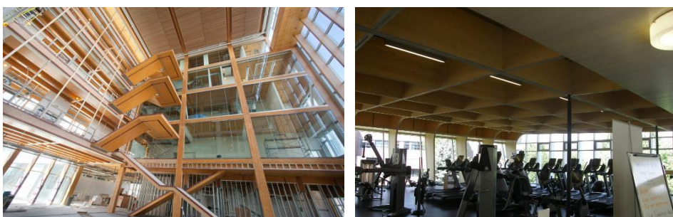
Figure 10: Wooden interior with CLT stairs (left), CLT frame and roof (right).
