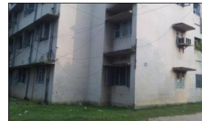
Figure 2(c): Staff Quater Building (No. 17)
