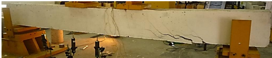
Figure 5: Failure mode of N1.9F RC beam
