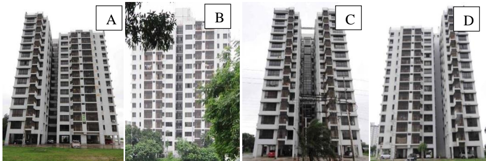
Figure 4: Elevation view of East (A), West (B), North (C), and South (D) (Source: Provided by MIST).
