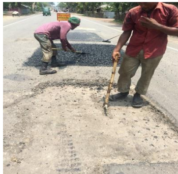
Figure 14: Top layer removed and re-filled by new asphalt materials
