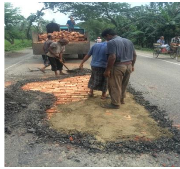
Figure 15: Brick soling and herring bone in N 5
