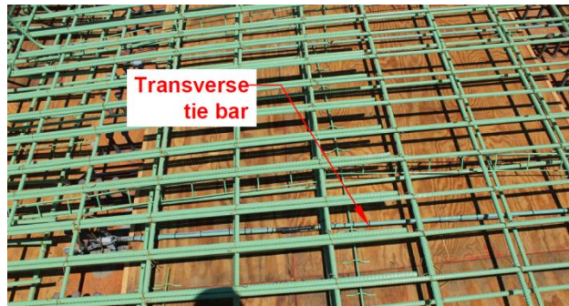
Figure 4: Transverse ties
