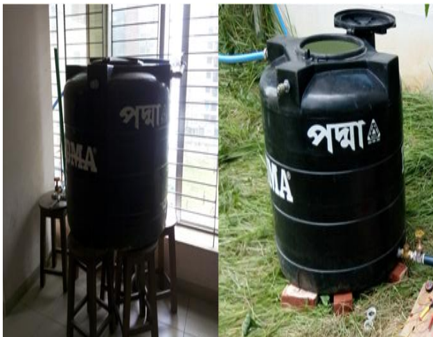
Figure6. Upper Tank (on 4 th floor) and Storage Tank (on ground)
