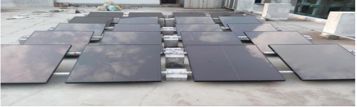
Figure5. Installed 2 KW Thin Film Solar PV Modules.
