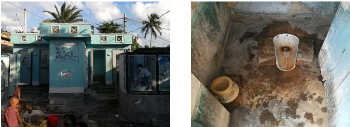
Figure 2: Bastuhara Community Toilet
