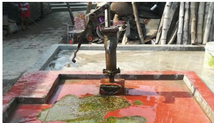
Figure 4: Tube-well (No. 6) used at Bastuhara Colony
