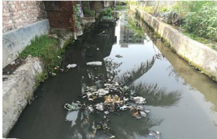
Figure 5: Existing Drainage Condition at Bastuhara Colony
