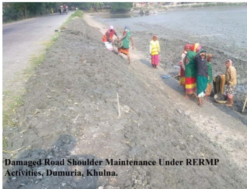
Figure 15: Mud dumping at side slope from dewatered fish farm (Location: Dumuria, Khulna)
