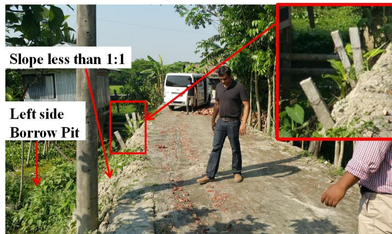
Figure 7: Steep side slope of rural roads in the study area (Location: Uttarpara, Uzirpar, Barishal).
