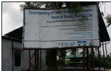
Co-compost plant at Baradi.
