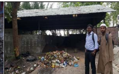
This compost plant has not capacity to manage whole wastes of the city.
