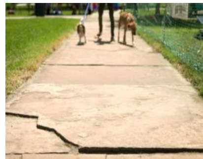
(b) Expansion Concrete Cracks
