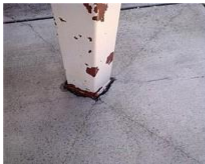
(a) Shrinkage cracks originating at re-entrant corners
