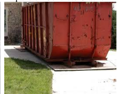
(e) Large Weights can Crack a Slab
