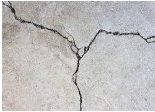
Crack on concrete structure
