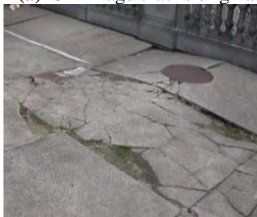
(c) Heaving concrete cracks
