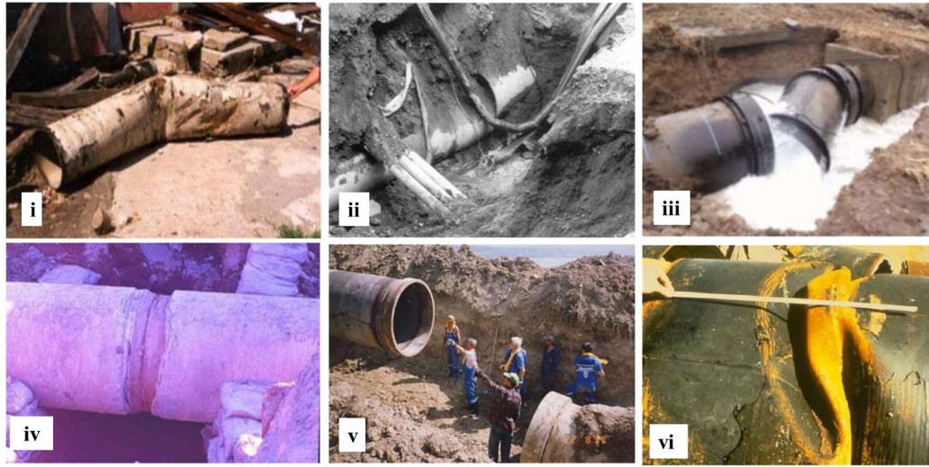
Figure 1-1: Examples of some earthquake induced buried pipeline failures due to: i) bending shell buckling of steel pipeline (1999 Kocaeli earthquake); ii) liquefaction-induced lateral spreading (1995 Kobe earthquake); iii) pullout of mechanical joints (2011 Tohoku earthquake); iv) Joint failure of concrete pipeline (1985 Mexico City earthquake); v) axial pullout of Asbestos Cement pipe (1999 Izmit earthquake); vi) axial shell buckling of steel pipeline (1971 San Fernando earthquake) [Gautam et al, 2018]
