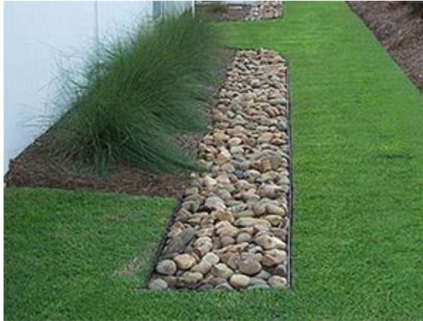
Figure 2.15 Pictures showing typical Infiltration trench (Wales, 2022)
