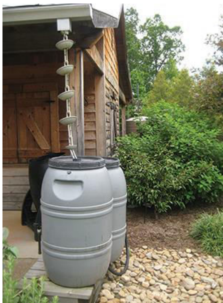
Figure 2.20 Picture showing typical Rain Barrel (adopted from Nebraska, 2022).
