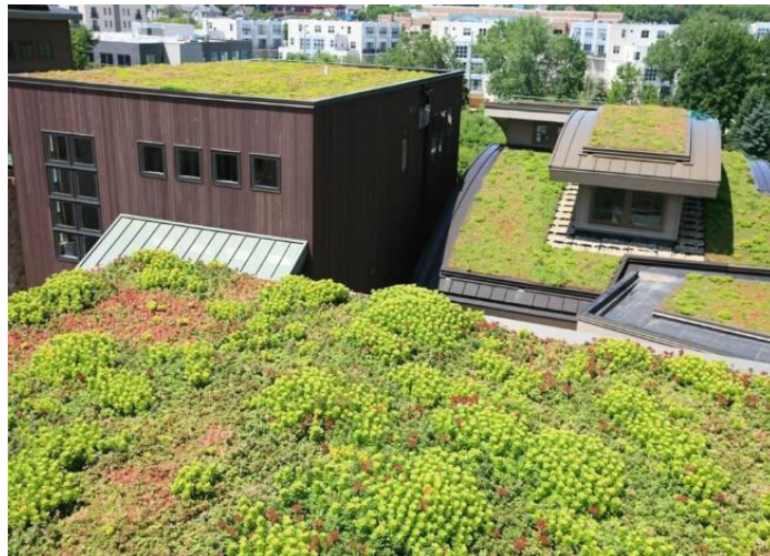
Figure 2.4 Pictures showing typical installed Green Roof system (adopted from LiveRoof, 2022).
