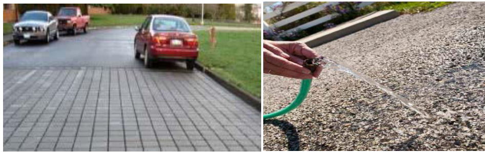
Figure 2.7 Pictures showing permeable pavement (adopted from Rossman, 1975).
