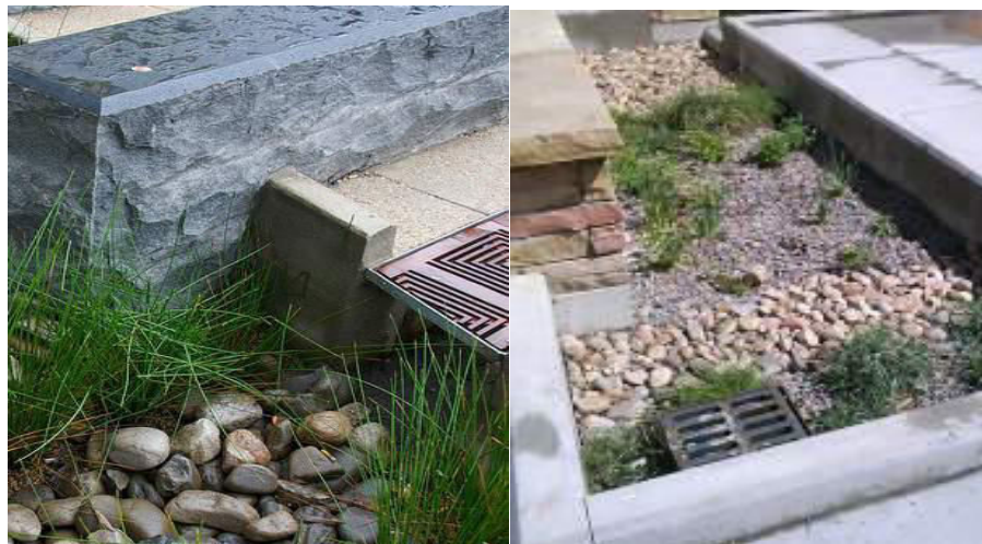
Figure 2.11 Pictures showing Bio-Retention Cells (adopted from Logan Simpson et al., 2015).
