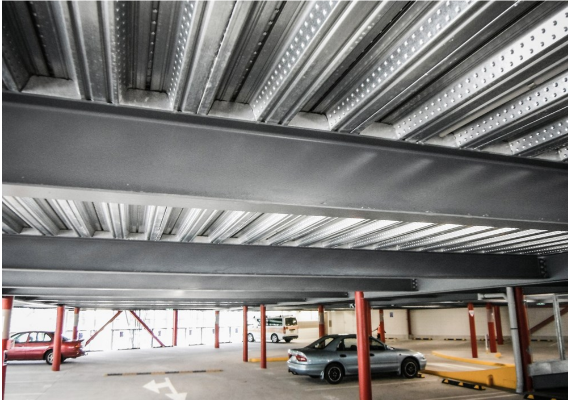
Fig. 1.1 Large Span Steel Concrete Composite Floor System [5]
