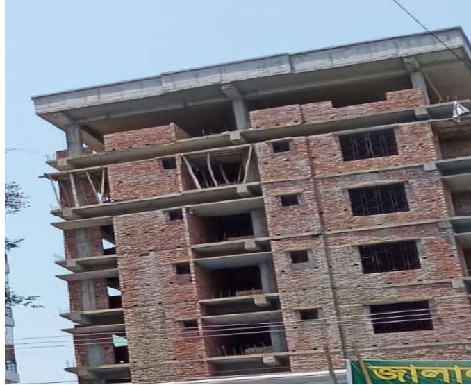
Figure 2-11: Masonry Units in a Typical Building of Chattogram City
