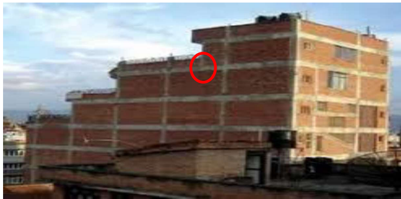
Figure 2-10: Building Vertical Discontinuities
