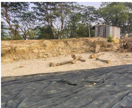
Damage road and vegetation due to Coastal erosion
