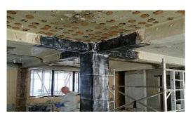
Fig. 8 Strengthening of Beam-Column joint using CFRP
