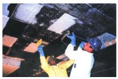
Fig. 4 Flexural Strengthening of Beam using CFRP sheet
