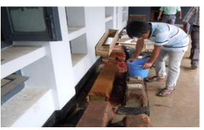
Fig. 2.2.3: Curing of beams
