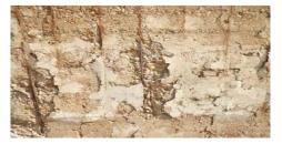
Fig 3: Deterioration of concretes in sewage treatment plant [Moradian et al., 2012]
