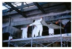
Fig. 3 GFRP fabric to strengthen deteriorated reinforced concrete T-beam
