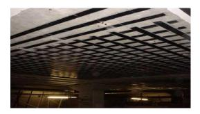
Fig. 7 Slab strengthening using CFRP laminates
