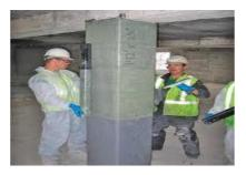
Fig. 5 Column confinement using carbon fiber sheet Fig. 6 Column strengthening using glass fiber sheet
