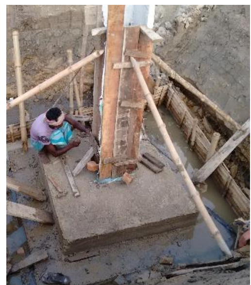
Fig. 4: (a) Section view- shallow foundation with reinforcement and (b) photograph of constructed shallow foundation with reinforcement in field
