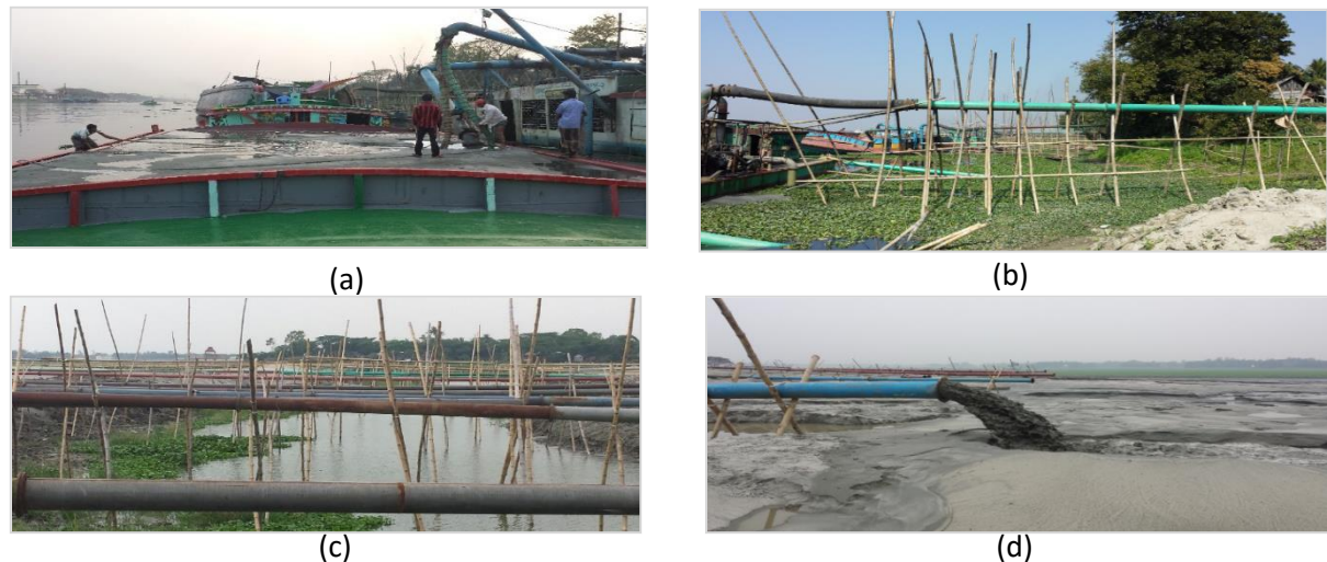
Fig. 1. Hydraulic filling procedure (a) dredged fill transported by barge (b) & (c) dredged fill transferred to the site in the form of slurry and (d) delivery of fill to the site.
