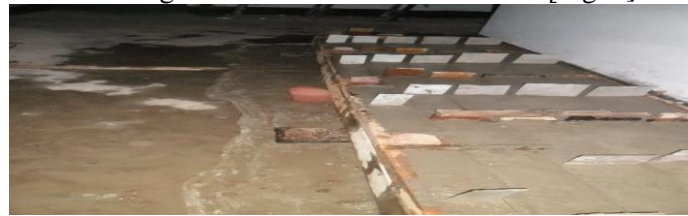
Fig. 1: Casting of pre-cracked beams inserting steel plates
