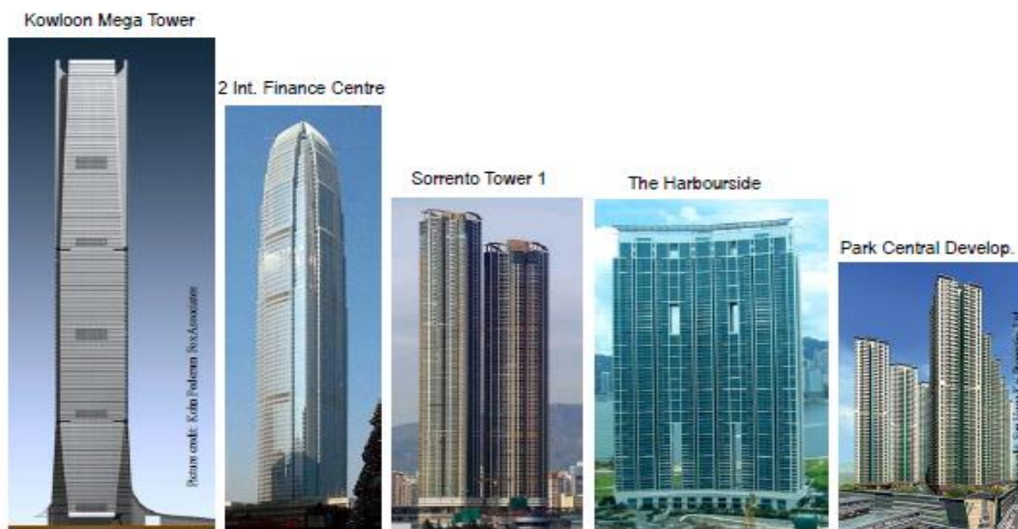
Fig. 1: Selected building projects optimized by OPTIMA in Hong Kong, China
