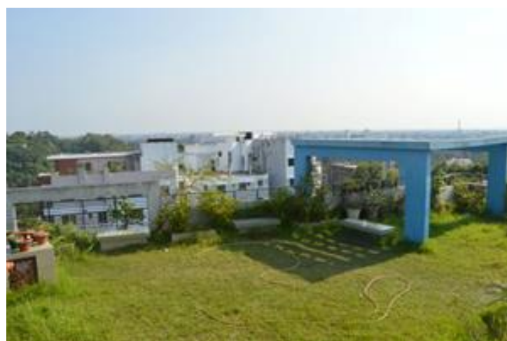
Fig. 3: Green roof application on the selected building
