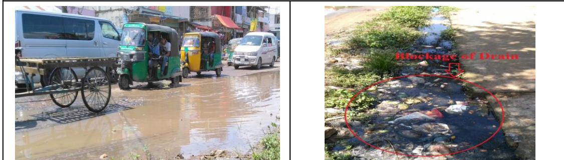
Fig. 2: Traffic problem & Blockage of drainage at Pahartali, Raozan, Chittagong.
