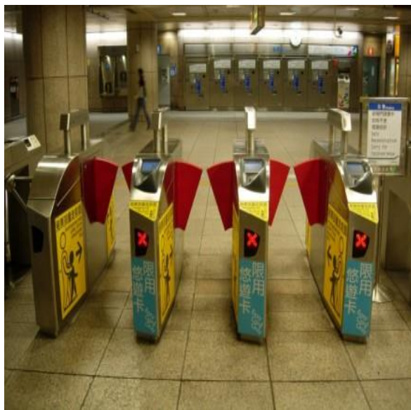
Fig. 7: Restricted entrance with rechargeable smart card system
