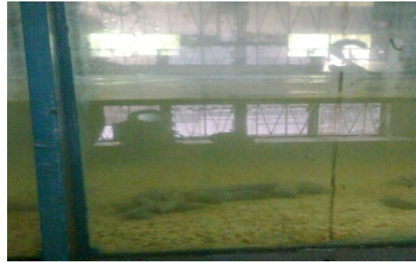
Fig. 4: Dumping of geobags
