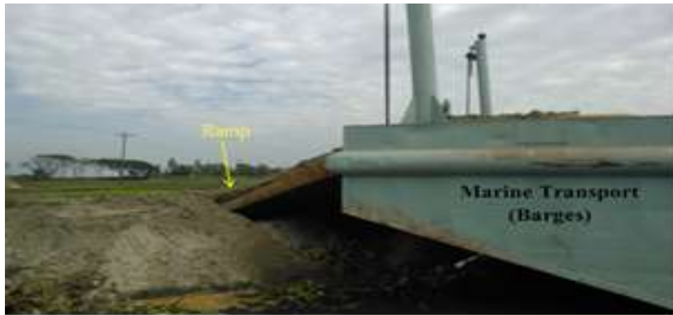
Figure 5(b). Rig unit unload arrangement from barges.
