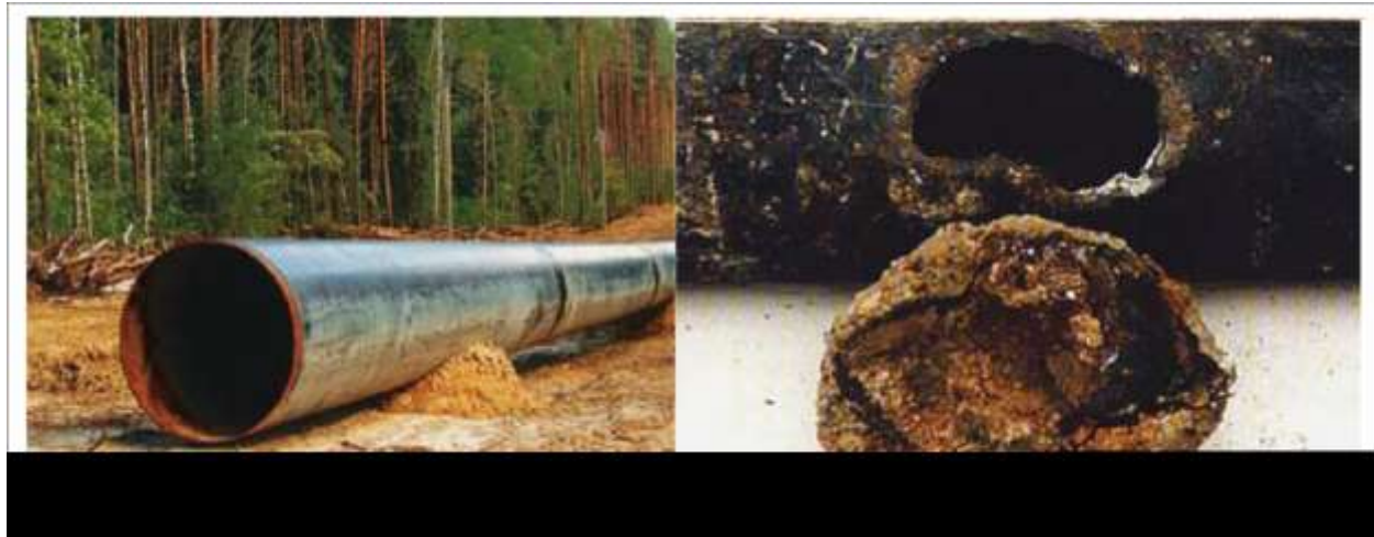
Fig 1: Leakage of pipe due to corrosion [39].
