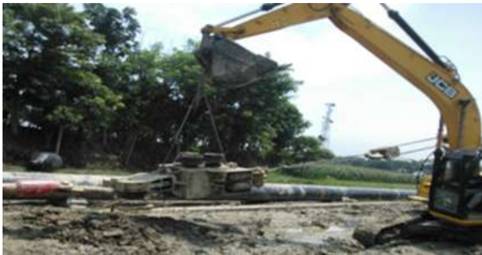
Figure 6(b). Vibrating hammer assembly at drill exit site
