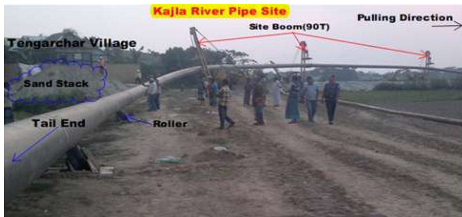
Figure 3 (a). Pipe pullback preparation at curve segment
