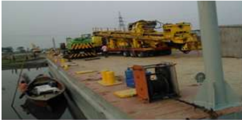
Figure.5 (a). Rig Unit mobilization by Barges
