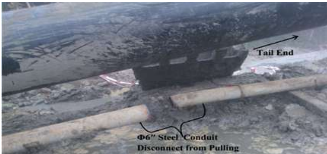
Figure 3(b). 6" Steel conduit disconnect from pulling head at kajla river
