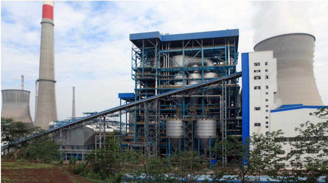
FIGURE 18 .The picture of operating 600MW SC CFB power plant.
