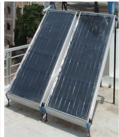
FIGURE 4. Solar water heater.
