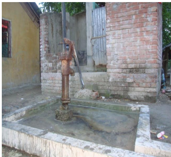
Figure 4: Unsafe distance between tubewell and latrine in Jogipole union
