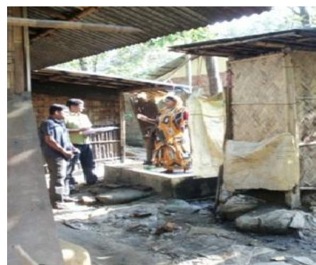
(b) Tubewell and latrine situated within 1-1.5 m , group 'A'
