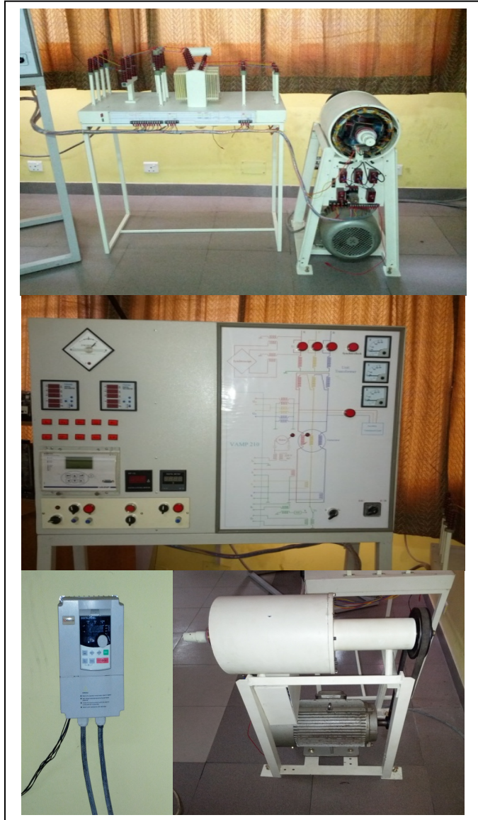
Figure 7: The complete schematic diagram of the generator protection project using VAMP 210 relay. First picture shows the Generator-Transformer unit, Second picture indicates the control panel for the fault clearing along with the entire block diagram of the system, 3 (right) denotes side view of generator along with the motor below which rotates the shaft of generator, 4 (left) Shows the Inverter system which is used to control the speed of the generator.
