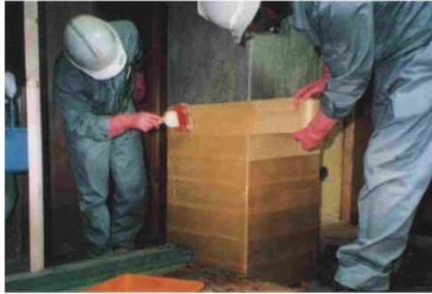
Fig. 4 Confining column with Aramid Fiber sheet (JBDPA report, 2005)
