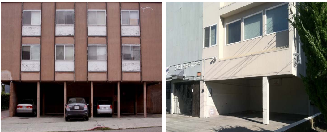
Fig. 1 Buildings associated with soft story (From Google image)
