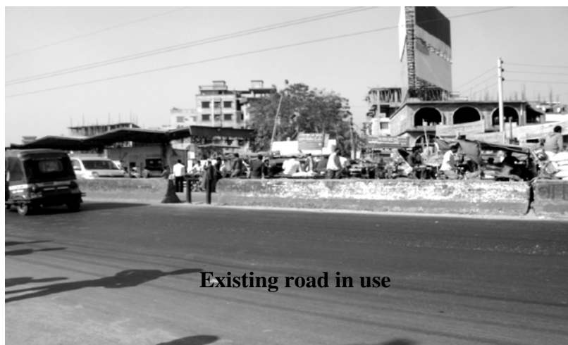
Figure: Existing Shanir Akhra-Jatrabari Road
