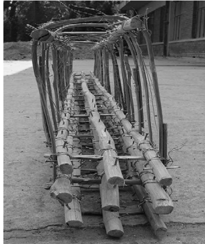
Figure 13: Alternately placed bamboo reinforcement
