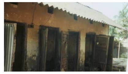
Figure 3: Community latrine (2007) in Kulibagan slum was unhygienic due to inadequate water.
