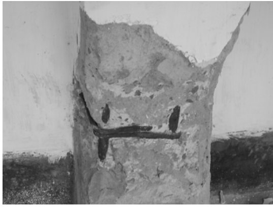
Figure 5: Plucking of old deteriorated concrete from column
