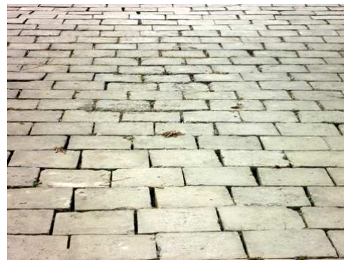
(b) CC block revetment
