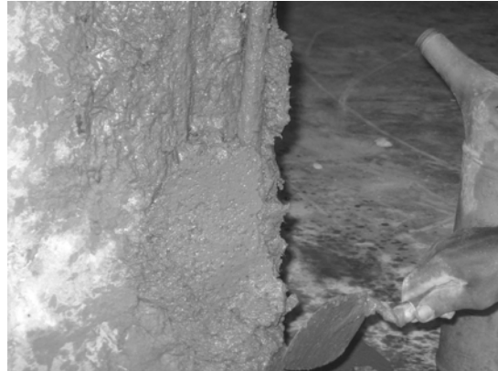
Figure 6: Rehabilitation of column by using nylon fiber
