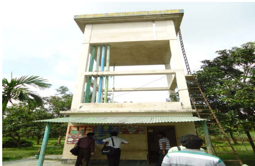
Figure 1: Water Supply Plant
