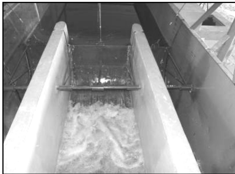
Figure 17: Nature of flow in the low Froude number stilling basin for the considered critical test condition
