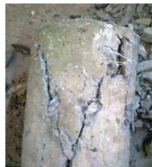
Figure 15: Wedge failure were observed in specimen C 2 and C 3
