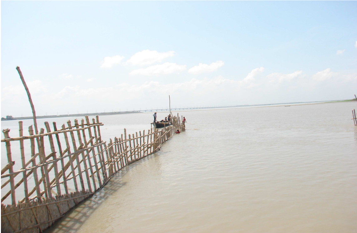
Figure 3: Bamboo Bandalling is going on in the Jamuna River of Bangladesh
