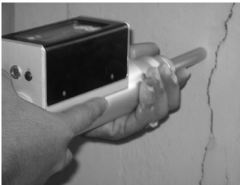
Figure 3: Non-destructive test of concrete by Schmidt hammer
