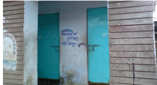
Figure 2: Renovated community latrine in Rupsha slum (2009), where community contribution was Tk. 1,455/= and ASEH grant was Tk. 7,029.
