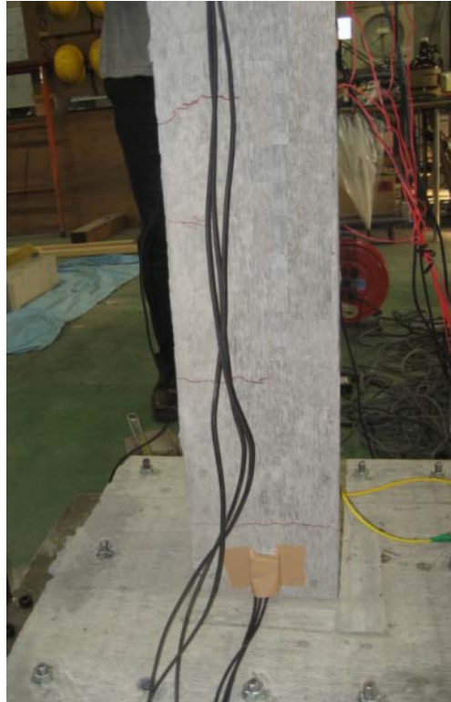
Figure 9: Test column after cracking
