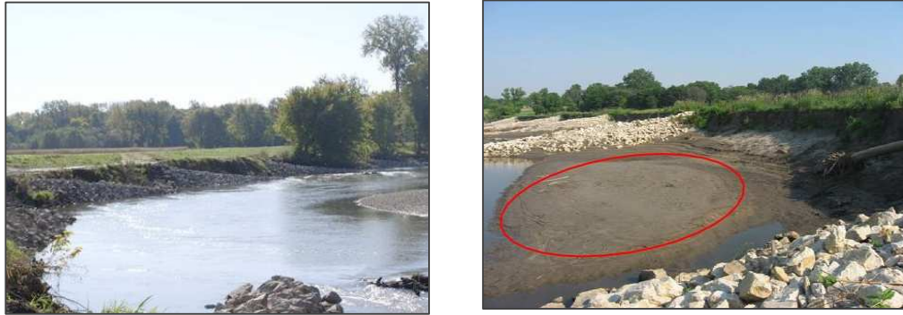
Fig.1. Photographic view shows the series of stream barbs installed along the riverbank during flow season (left side) and low flow season (right side). The red circle indicates sand bars formed after installation of barbs.
