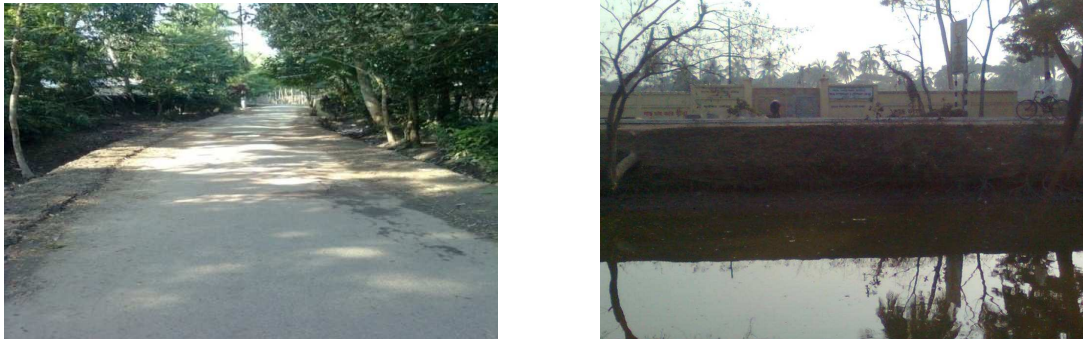
Fig. 4: Present embankment system in beel dakatia (Raghunathpur, March, 2011)
