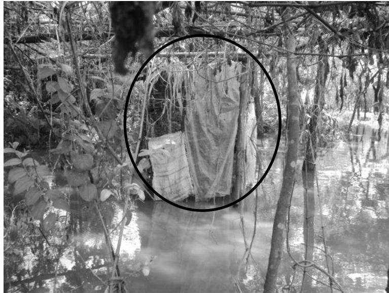
Figure 6: A common feature of pit toilet in waterlogged area
