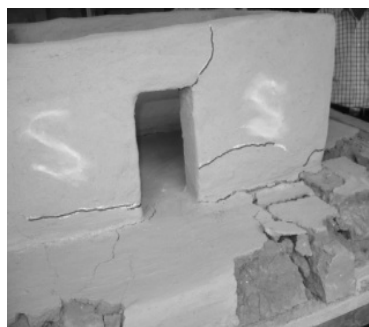
Figure 13: Position of crack formation in unreinforced mud house in experiment.
