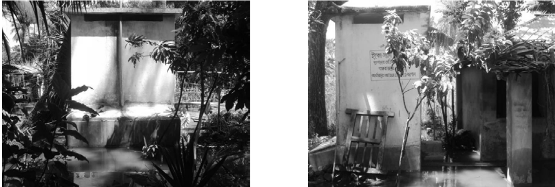
Figure 8: Ecosan toilet in waterlogged area
