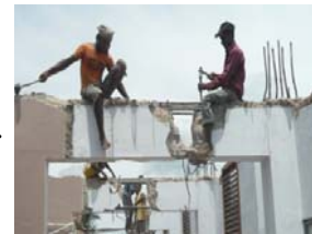
Fig 5d: Demolition of R.C.C beam
