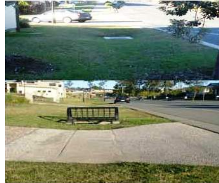
Figure 5: Swales with various inlets
