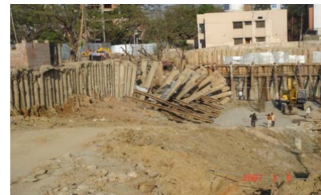
Fig 4. Failure of shore piles in Basundhara
