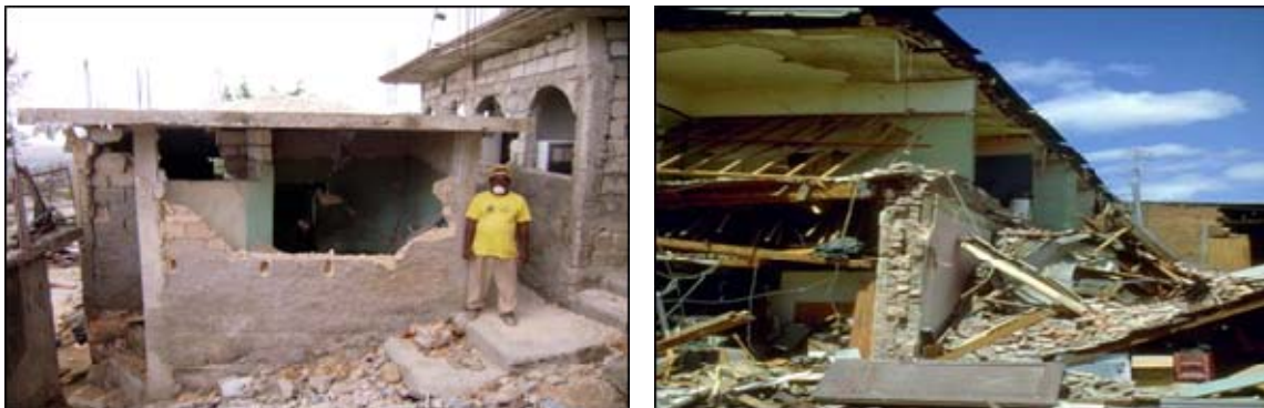
Fig. 4: Significant damage of structural masonry in (a) Haiti (2010) (b) California, USA (1981)
