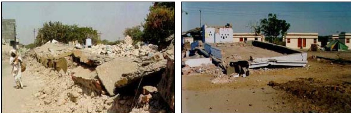
Fig. 3: (a) Total collapse of masonry building, (b) Lintel band preventing collapse (Bhuj 2001)
