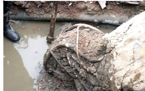
Fig 12. Buckling of north-east corner column
