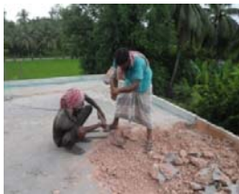
Fig 5a: Demolition of lime terracing layer
