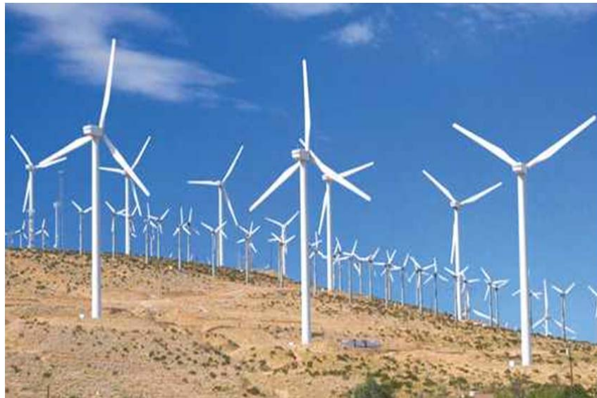
Fig. 8: Placement of Turbines
