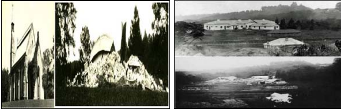
Fig. 2: Collapse of masonry (a) All Saints Church, (b) Girls School in Shillong (Assam 1897)
