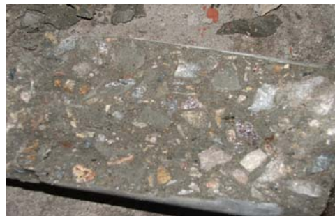
Fig-5 (a): Normal concrete after failure
