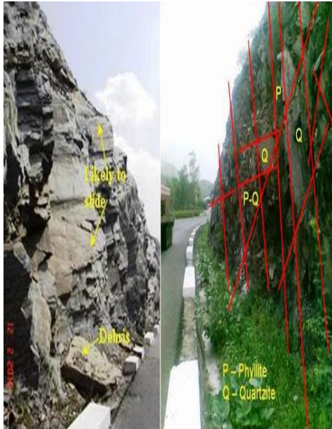
Fig 6: Roadside hill cut slopes NH-8 between Udaipur-Ahemdabad
