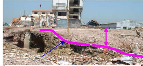
Fig 11. Settlement of NE corner of GF
