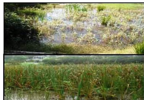
Figure 6: a. Bioretention Water Logged b. Three Years After Maintenance.
