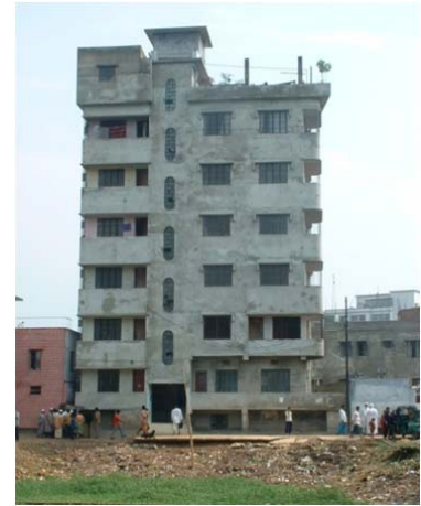
Fig 2. Eight storied building at Mirpur tilts
