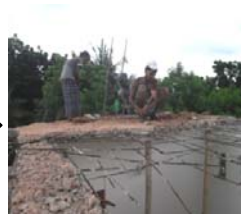
Fig 5b: Demolition of R.C.C slab
