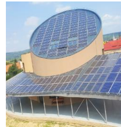
Fig. 5: Photovoltaic system on grid system 60 KWp.
