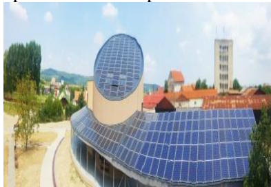
Fig. 5: Photovoltaic system on grid system 60 KWp.
