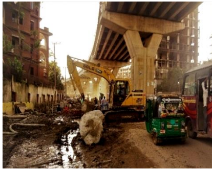
Fig. 6: Closure of roads and footpaths
