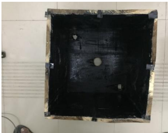
Fig 7.3: Inside wall of the box
