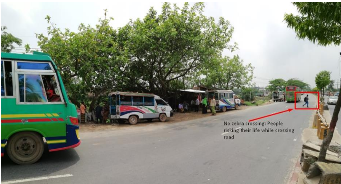
Fig. 2: Road crossing problem in Boliarpur Bazar (Dhaka-Aricha Highway)
