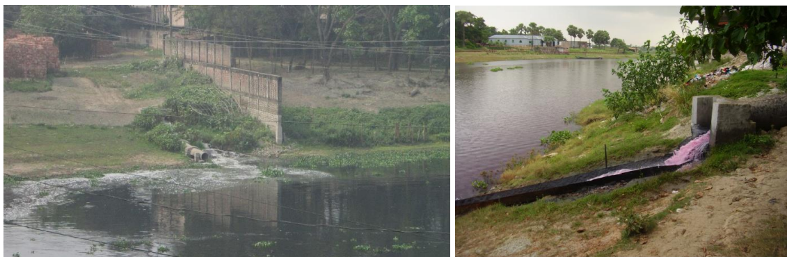
Figure 3: Sewerage water and Industrial waste water falling into river
