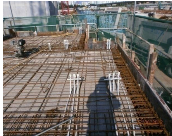
Figure 15: Top layer of rebar placed and slab is ready for casting
