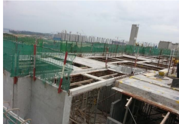
Figure 13: Preparation for precast plank placement
