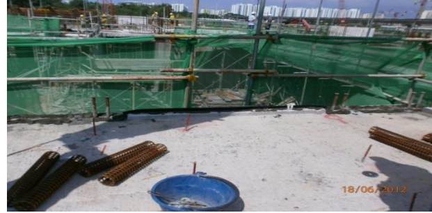
Figure 9: Bedding preparation for façade installation
