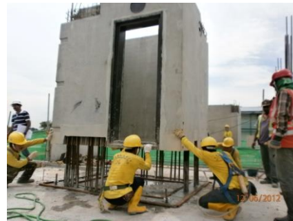
Figure 23: High quality workmanship using PPVC
