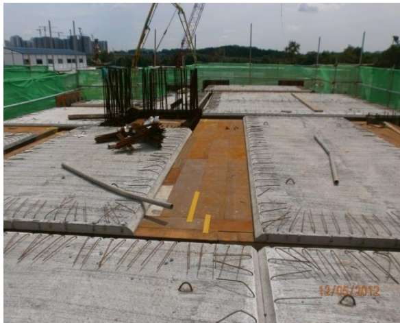
Figure 14: Placing of precast plank
