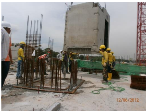
Figure 18: Installation of household shelter in progress
