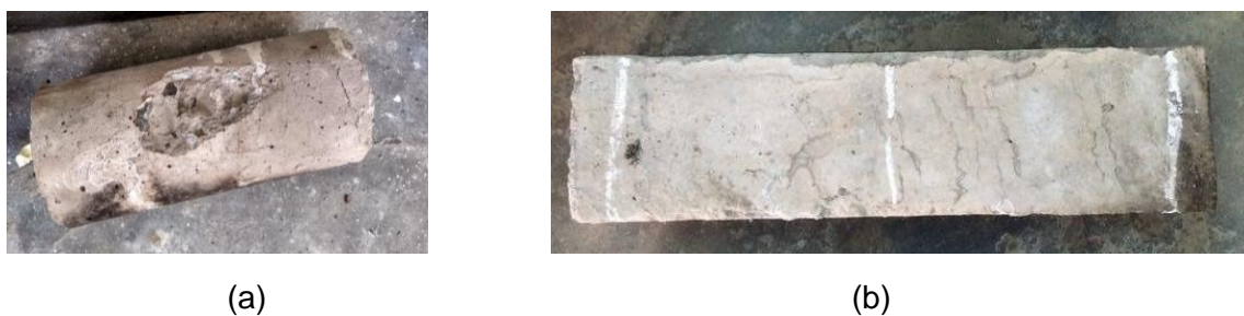
Figure 4: Spalling and cracks in specimens; (a) spalling in cylindrical specimen, (b) cracks in beam specimen.
