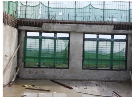
Figure 11: Façade panel being installed
