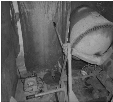
Figure 1: Mixing of Concrete
