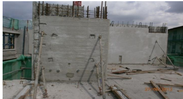
Figure 7: Column after installation of column wall connection
