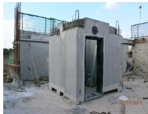
Figure 19: After installation of household shelter
