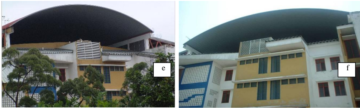
Figure 1: Field application of profiled steel sheet for roofing system
