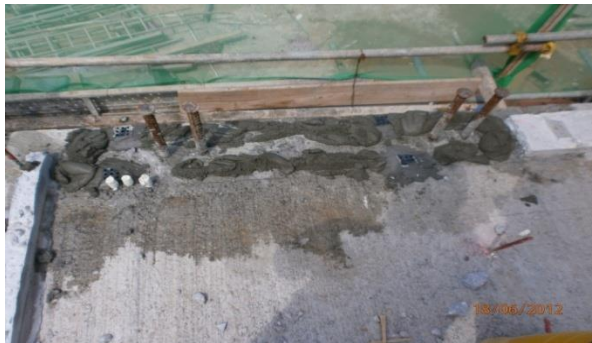
Figure 6: Bedding preparation for column or wall connection
