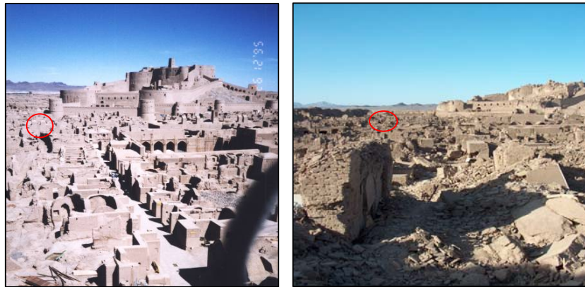
Figure 1 Pyambar Mosque before and after the earthquake of December 2003
