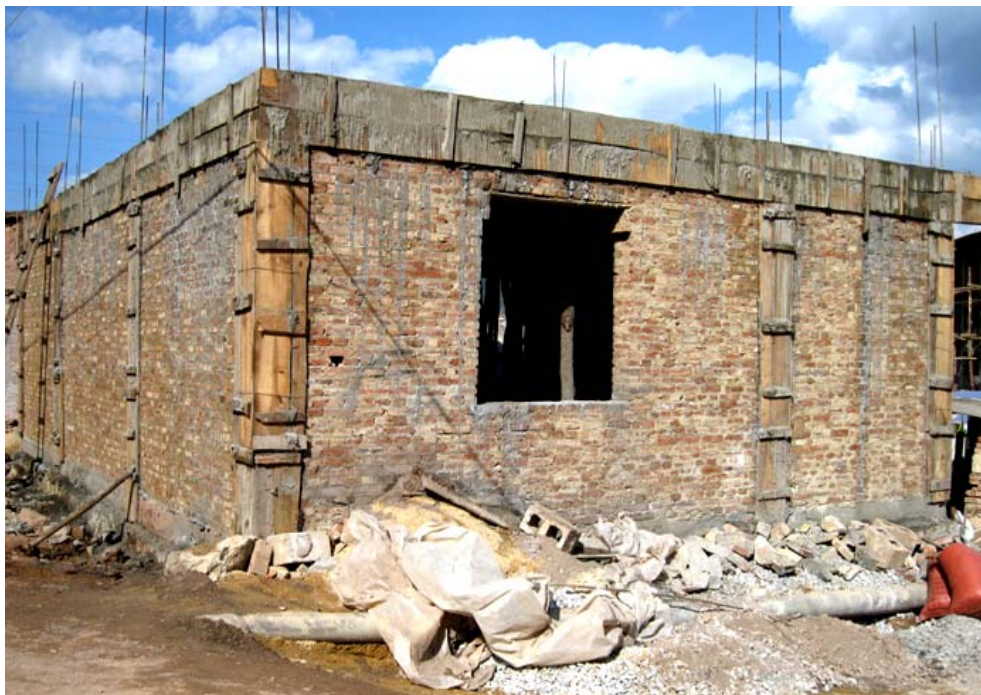
Figure 5 A typical brick-concrete structure building in Yunnan Province
