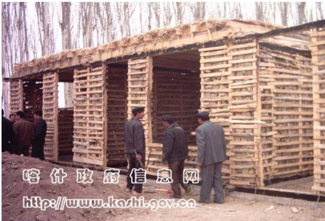
Figure 3 A building with a wooden sandwich structure in Xinjiang Uigur Autonomous Region
