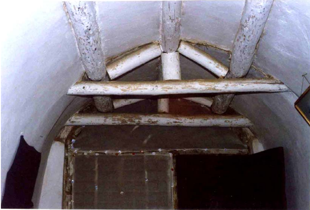
Figure 4 A simple anti-seismic structure for cliff kilns
