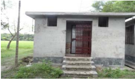
Figure 3: Super structure of the biotoilet (under construction)
