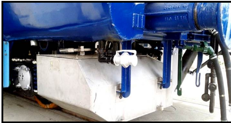
Figure 2 Bio Toilet System in Train
