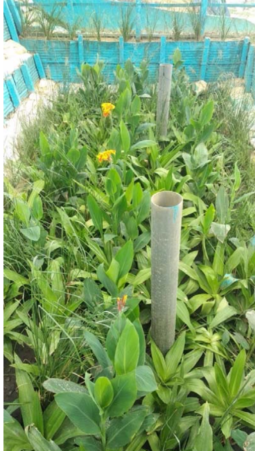
Figure 3: Different types of plants are used in FSM treatment plant (constructed wetland unit)
