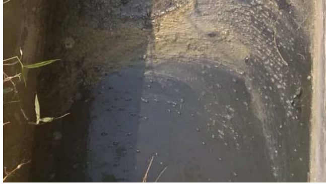
Figure3Condition of the observed drain.
