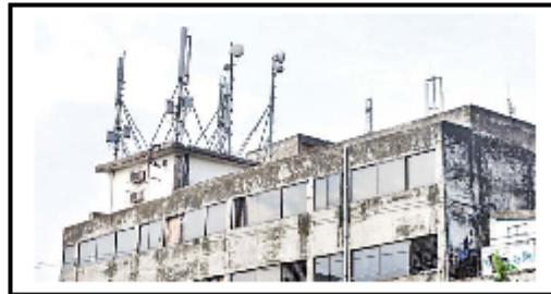
Fig. 1. BTS established at the rooftops of buildings [15]
