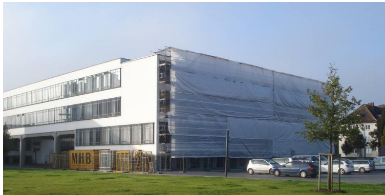
Fig. 4. Bauhaus building during renovation, © Winfried Brenne Architects
