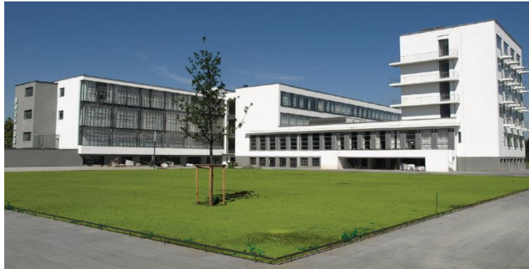
Fig. 1. Bauhaus building Dessau, © Winfried Brenne Architects
