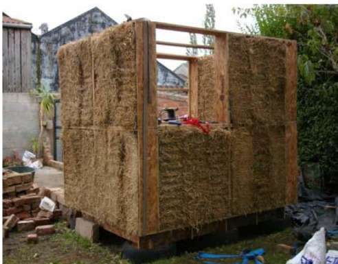
Fig. 1. Erection of test rig blocks
