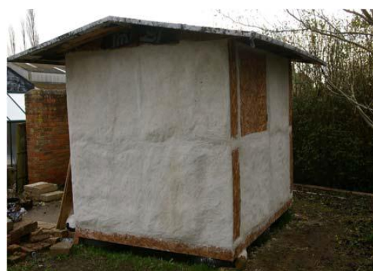
Fig. 2. Completed rig construction
