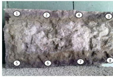
Fig. 4. Measuring chloride penetration depth
