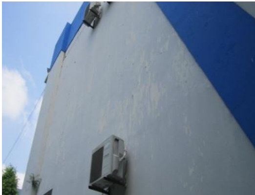
Fig. 1. Paint chipped walls.
