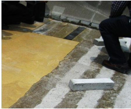
(a) Mortar grout applied during 1 st trial repair work.
