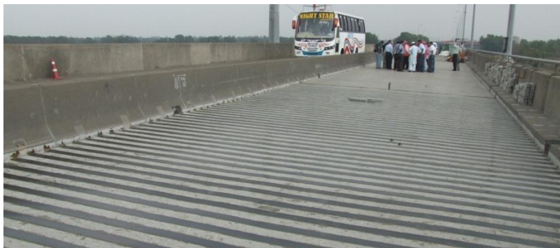
(e) CFRP strips laid across the carriageway.
