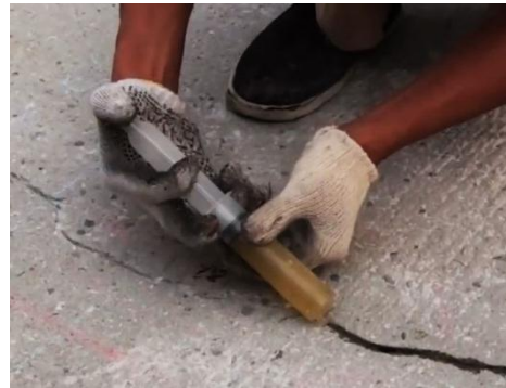
(b) Filling the grooves with epoxy.
