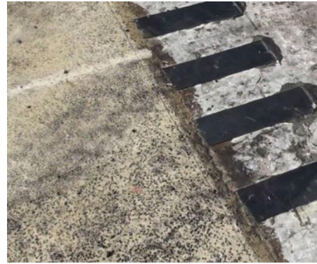
(b) Mortar grout overlaid by scattered stone chips in actual repair.
