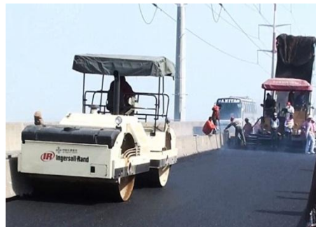
(b) Paving the carriageway with 50mm thick SMA.
