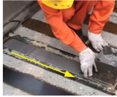
(b) Laying epoxy over primer by sliding the mould.
