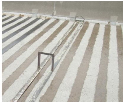
(a) Strips of epoxy primer applied.
