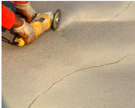
(a) Groove cutting along the cracks
