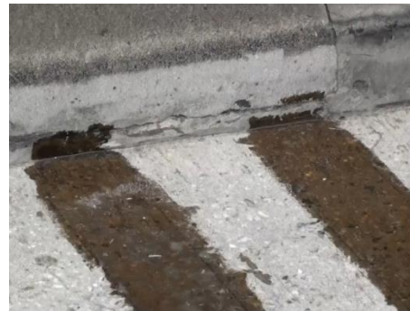
(b) Close-up view of epoxy primer strips.
