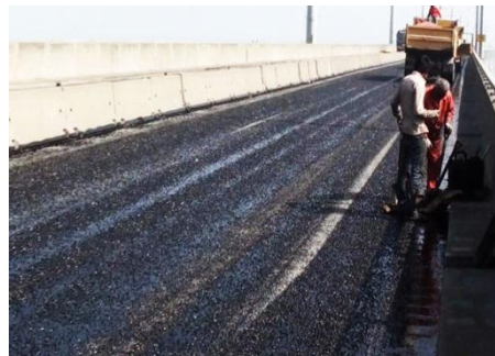
(a) Epoxy asphalt water proofing membrane applied on mortar grout.
