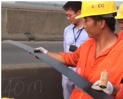
(c) A CFRP strip is being taken to place.
