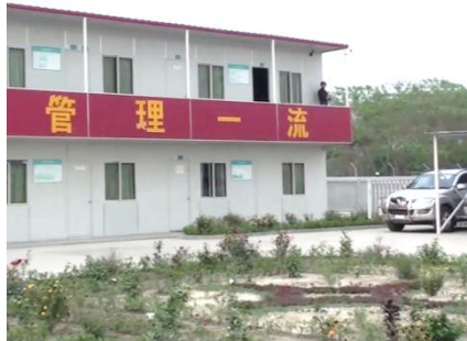
(a) CCCC site office and laboratory.
