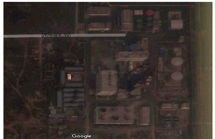
Fig. 3: NWPGL 230kV substation near the proposed land
