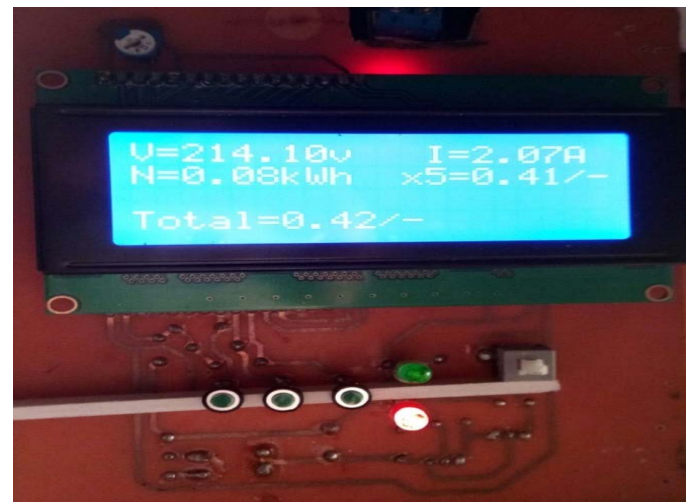
Fig. 4. Practical implementation of Normal Mode in Dual Mode Energy Meter ('N' stands for Normal Mode)
