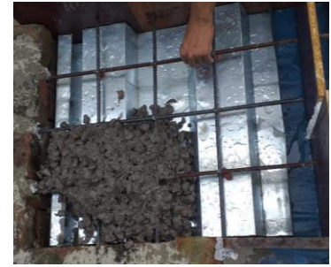
Fig. 7: Concrete placement
