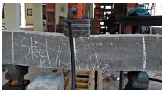
(b) Cracks in 1.5% steel fiber beam
