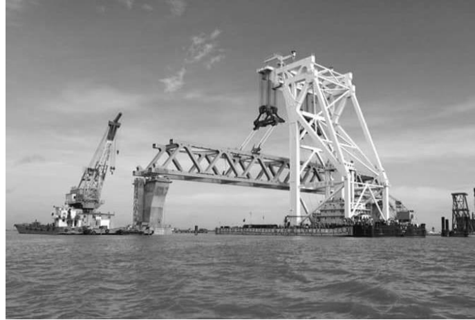
Figure 2: Intallation of Span (www.padmabridge.gov.bd)
