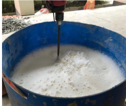
Figure 1: Mixing procedure of foamed concrete
