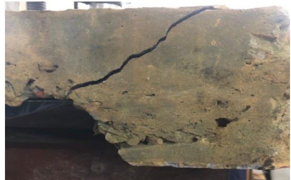
Fig.11: Crack propagation of slab under loading
