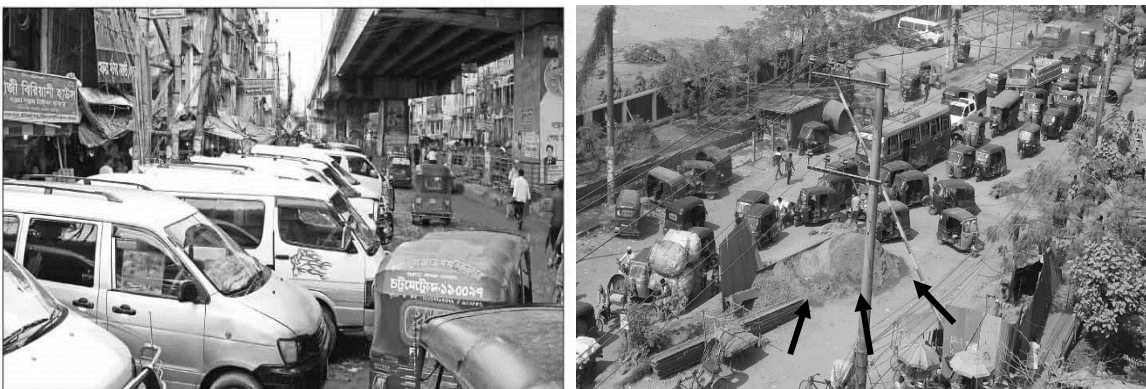
Figure 2a, 2b: Traffic mismanagement due to illegal parking and construction materials on road
