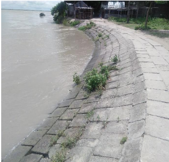
Figure 4: Primary stage of CC Block, Shuressor, Shariatpur District (15 November 2000)
