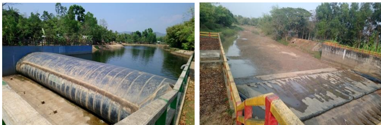
Figure 2: Menongchara and Buraghat rubber dam
