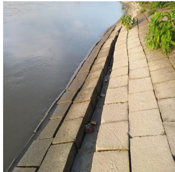
Figure 5: Final stage of CC Block, Shuressor, Shariatpur District (15 November 2006)
