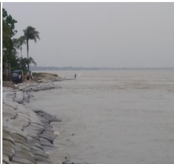
Figure 3: Final settlement of Geo Bag Filling Chandipur, Shariatpur district (05 March 2001)
